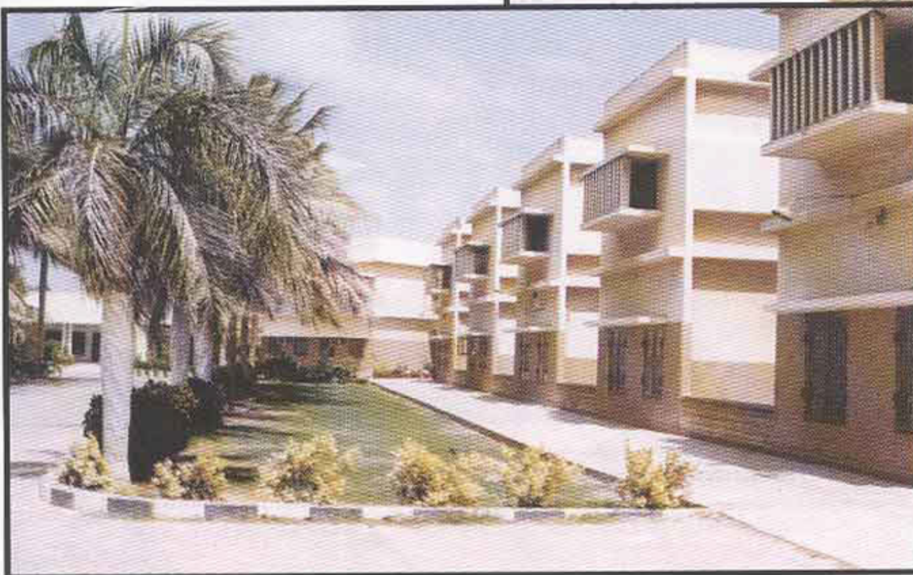
Some administrative offices and consultation room, a photographic view
